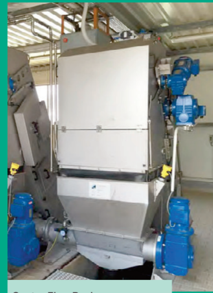
Center Flow Rechen
