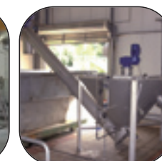
▲ Grit washer unit
