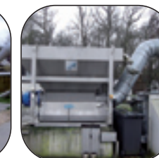
▲ Septage receiving Station FK 100
