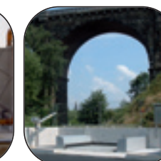
▲ Grit receiving station
