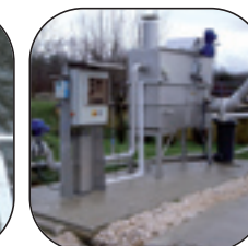
▲ Compact screen/Septage receiving station
